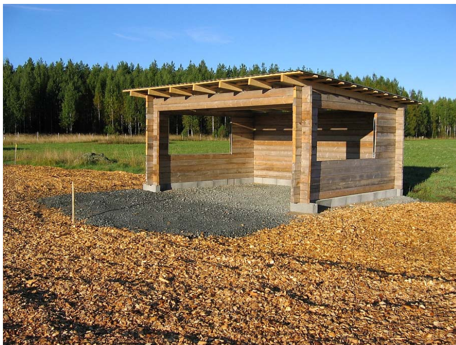
Fig. 3. Weather shed built at Kuuma. In the foreground the paddock area with wood chips can be seen. Note the crushed stone powder area in the front of the shelter (photo Aaro Närvänen).
