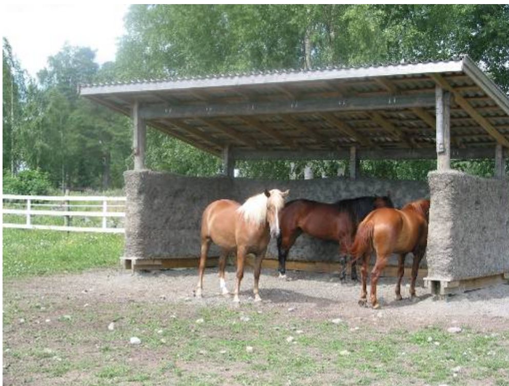
Fig. 2. The clay-straw weather shed built at the Equine College Ltd, Ypäjä in summer 2007 (photo Helena Jansson).
