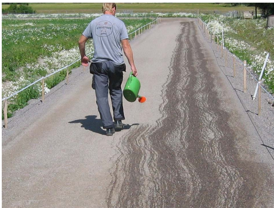
Fig 4. Spreading ferric sulphate solution on the Kuuma oval track (photo Aaro Närvänen).
